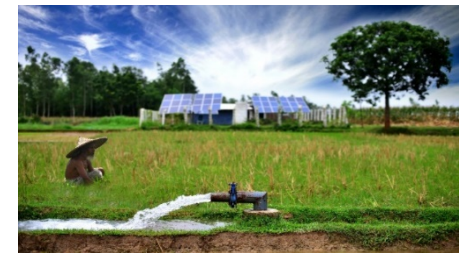
Solar irrigation Pump
