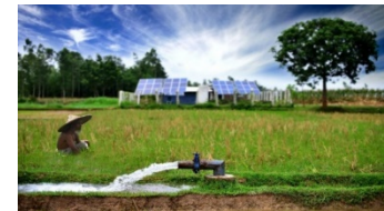
Solar irrigation Pump
