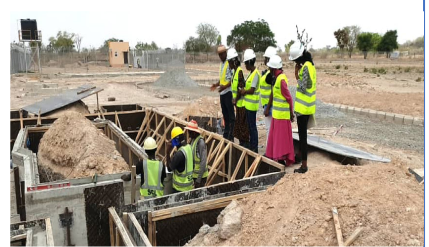
Training on casting foundations
