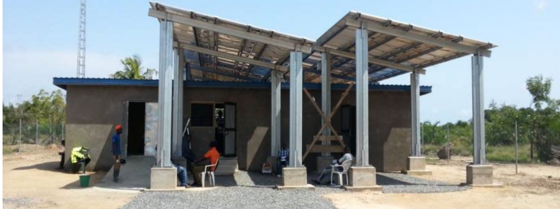
GENERATION SUB-SYSTEM – SOLARPV/ WIND & DIESEL GENSET BACKUP HYBRID SYSTEM @ Perdiatorkope
