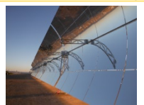
CSP Parabolic Trough
