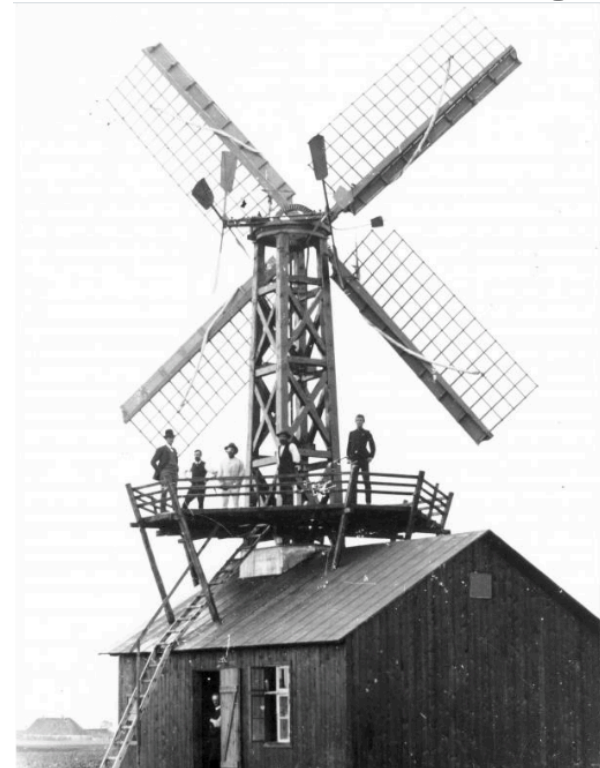
Denmark's first electricity-producing wind turbine was built at Askov University College in 1891 with a rotor diameter of 11.6 meters. It is the inventor, Poul la Cour, who peeks out from the engine house under the mill. The other people are the craftsmen who built the wind turbine. (Illustration: Poul la Cour Museet)
