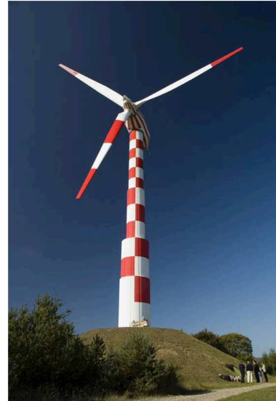
Tvindkraft wind turbine near Ulfborg Denmark in northwestern Jutland. The 60-meter diameter wind turbine has operated since 1979. At the time of its installation it was the largest wind turbine in the world. There is an exposition on the construction of the turbine in the base of the concrete tower.
