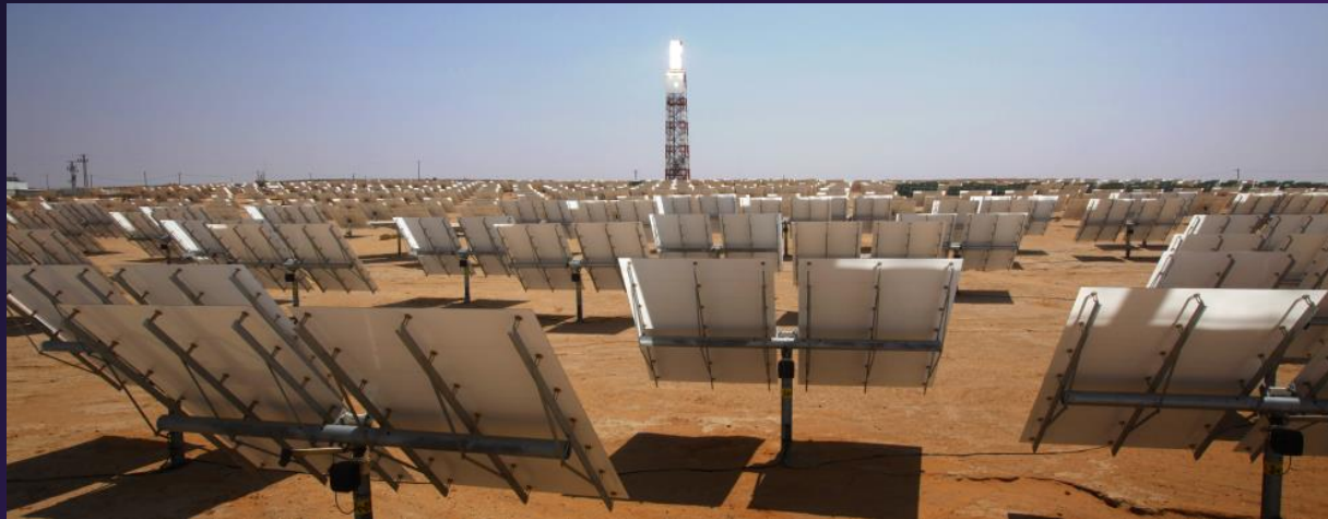
In a CSP system with thermal energy storage, the heat transfer medium, such as molten salt, retains heat so well that it enables the plant to generate electricity for hours when the sun is not shining.
