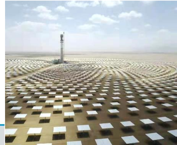
In a CSP system with thermal energy storage, the heat transfer medium, such as molten salt, retains heat so well that it enables the plant to generate electricity for hours when the sun is not shining.
